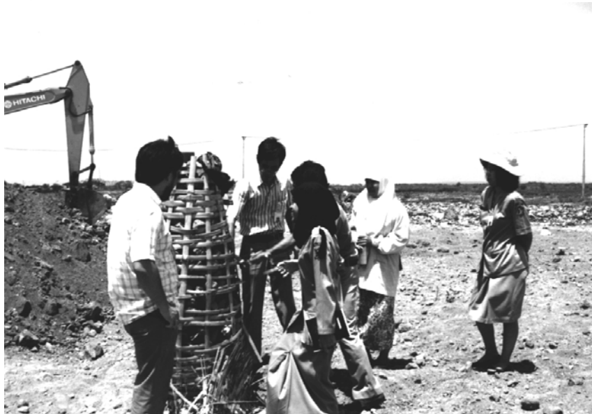
Picture 3.3 Gas venting cage made of bamboo in Indonesia (JICA Study 1992)
