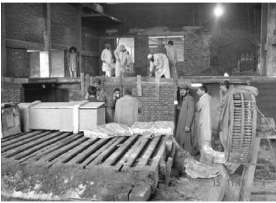
Fixing New Furnace
